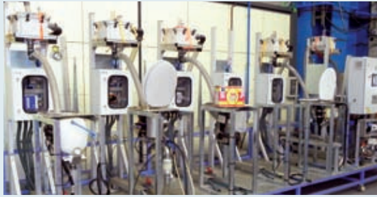
The test bench is installed at Alstom's Barcelona plant.
